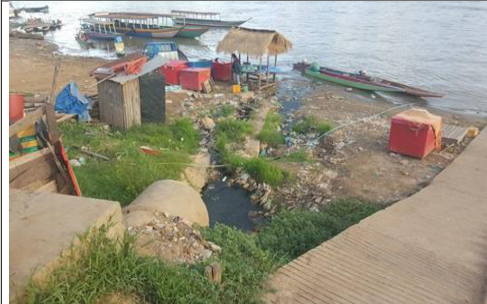
Figure 25b: Nakasang grey water drainage discharge into the Mekong to be extended
