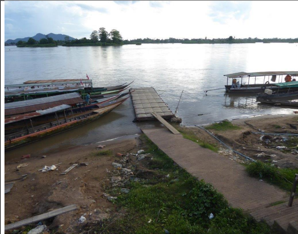
Figure 11c: Existing floating pier & pedestrian ramp to be improved.
