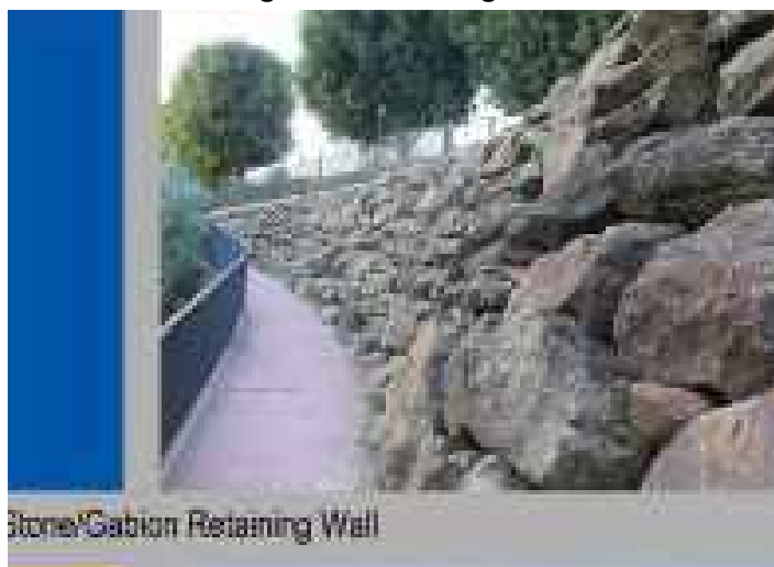
Figure 8: Retaining wall
