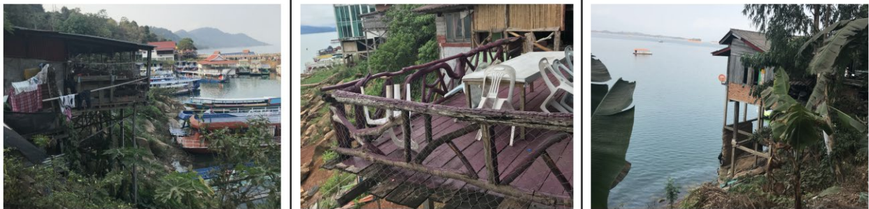
Figure 2: Current Structures Along Shophouse Road
