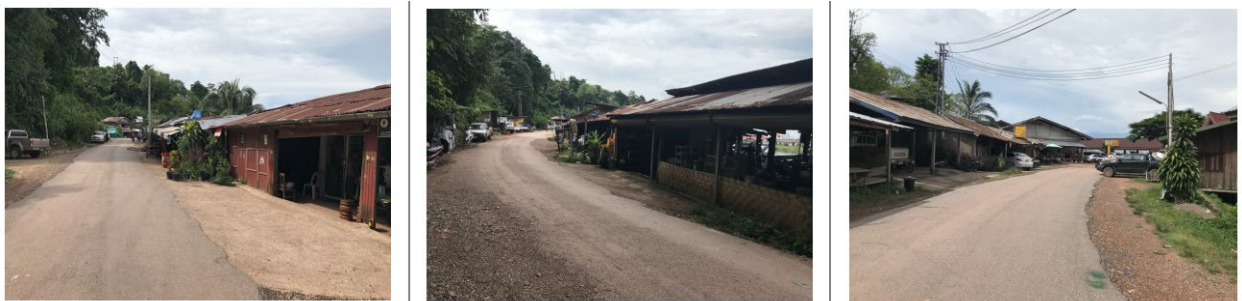
Figure 3: Shophouse Road – View South to North
