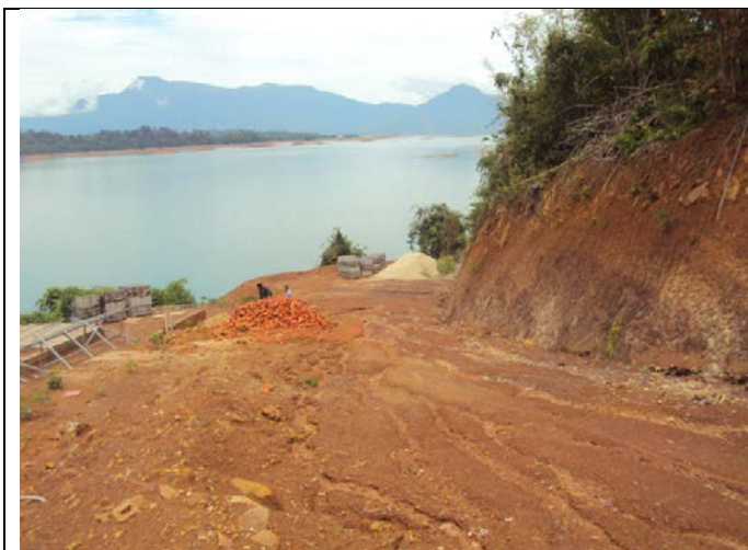
Part of site for new road construction and upgrading
