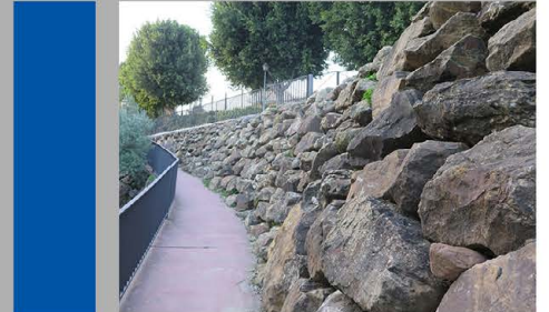
Stone/Gabion Retaining Wall
