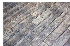
Wood plank pattern stamped concrete
