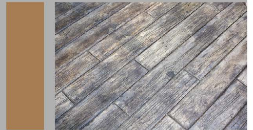
Wood plank pattern stamped concrete
