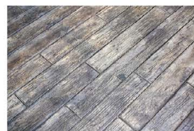
Wood plank pattern stamped concrete
