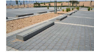
Concrete Car stopper
