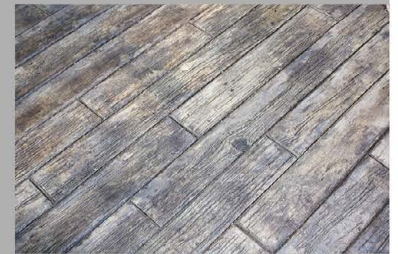
Wood plank pattern stamped concrete
