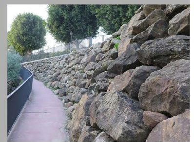
Stone/Gabion Retaining Wall
