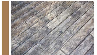
Wood plank pattern stamped concrete
