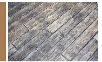
Wood plank pattern stamped concrete
