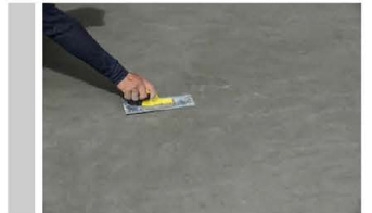
Concrete trowel finish
