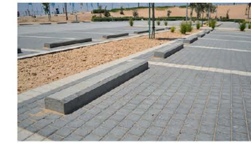
Concrete Car stopper
