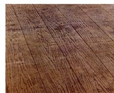
Wood pattern stamped concrete
