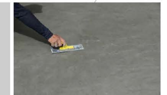
Concrete trowel finish
